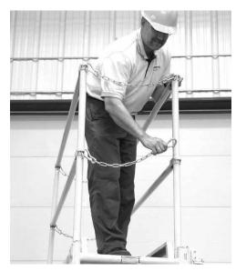
7. Adjust base outriggers to maintain a 3:1 height to base ratio in keeping with applicable legislation. Always engage the outrigger latch pin before climbing the Tele-Tower.
