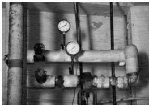
Pipe insulation
