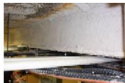
Thermal Sprayed-on Insulation
